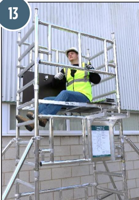
13. Fit 2 guardrail frames, with the top hook (facing outwards) set above the top rung of the frame.
