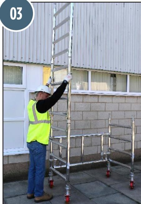
3. Connect 2 frames together and fit onto the base section at each end.
