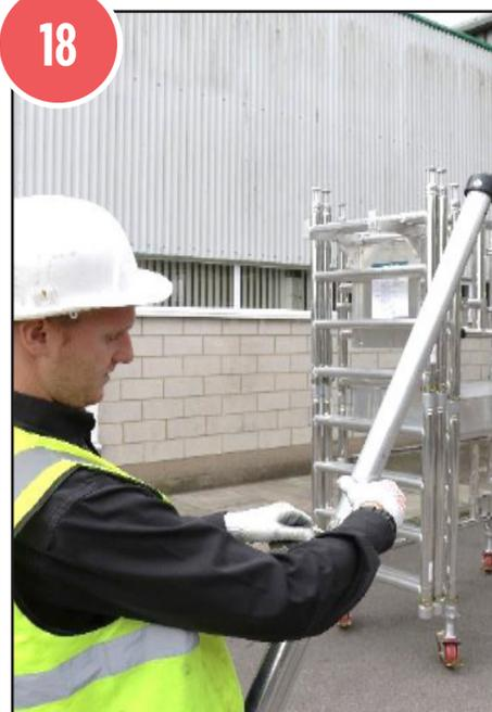
18. Before fitting stabilizers, release the pin to enable extension.
