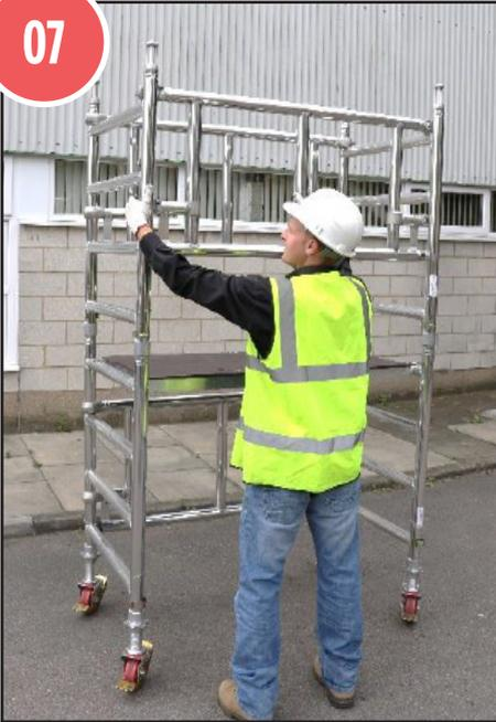
7. Fit a guardrail frame to each side of the platform (hooks facing outwards) Top hook above the top rung of the end frames. (Refer to labelling to ensure that the frame is the correct way up).
