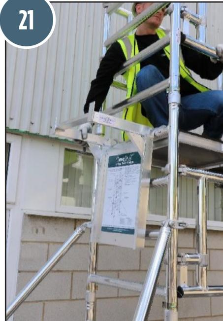
21. Relocate the "empty" assembly bracket from the side of the tower.
