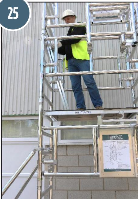
25. Temporarily locate the toeboard assembly on the platform to allow access to the additional platform that is stowed.
