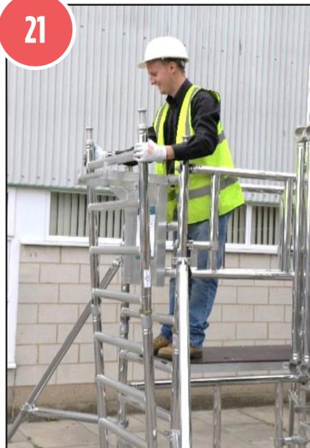
21. Retrieve a set of frames from the side assembly bracket and fit.
