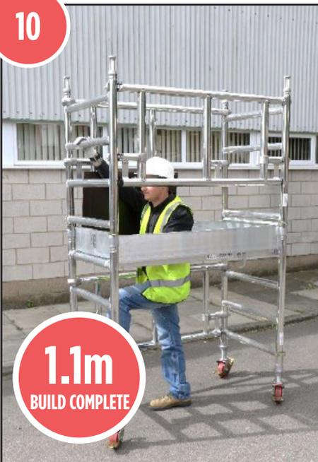
10. Access the platform using the trapdoor as shown and begin work.
