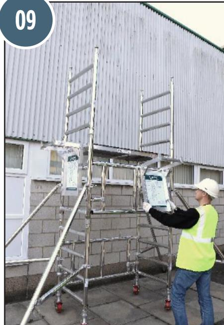
9. Fit the additional assembly bracket on the front of the tower as shown.
