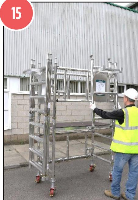
15. Stow 3 guardrail frames on the front assembly bracket.
