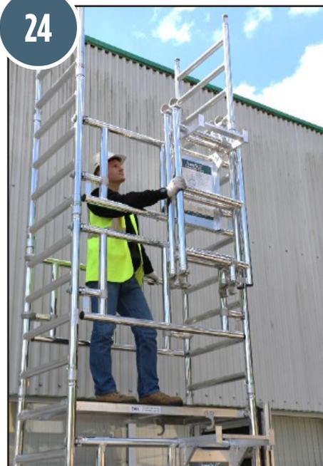
24. The frames are relocated as shown.
