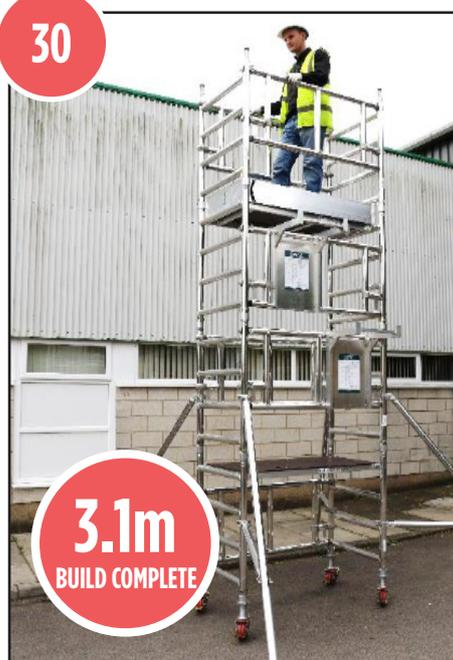
30. Access the platform using the trapdoor and unfold the toeboard.
