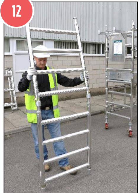
12. Assemble the frames in pairs as shown.
