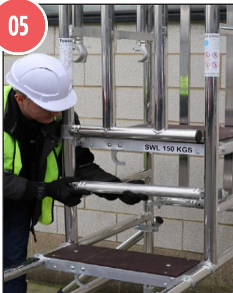
When building the Stepfold 2 add a ribbed brace below the platform.
