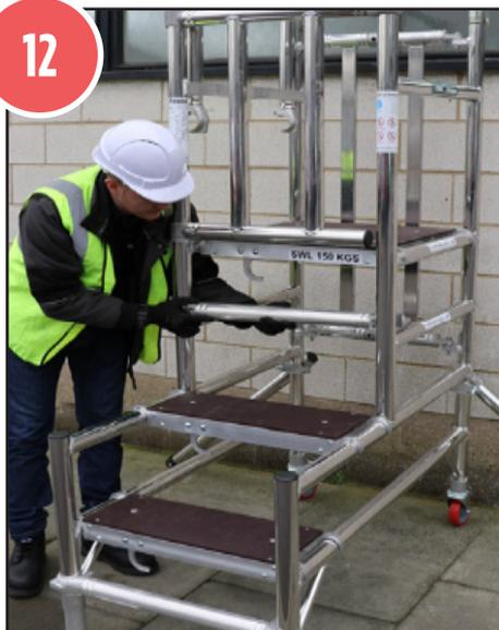
Add the additional brace below the platform. For a stepfold 2 you should now have 2 ribbed braces below the working platform.
